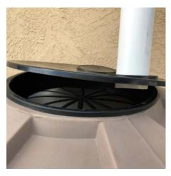
Next, locate the overflow extension screen (1) for your tank. Install it onto the tank overflow fitting (2) by pressing it on.
